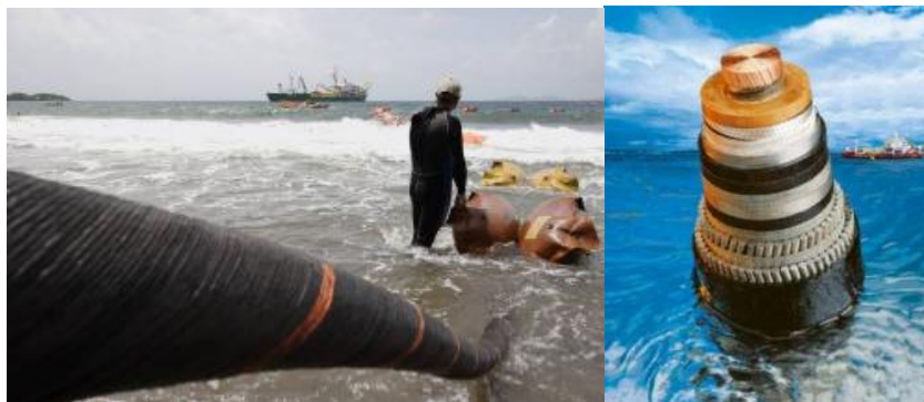
Laying of the HVDC cable
